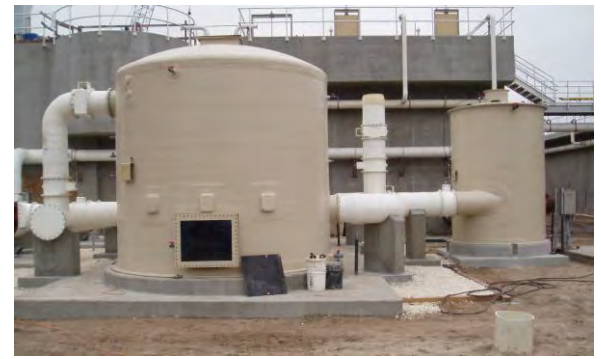
ECS designed and manufactured radial flow carbon polishing unit
